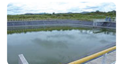
Bridgestone Carbon Black (Thailand) Co.,Ltd. (BSCB)の雨水貯留池
